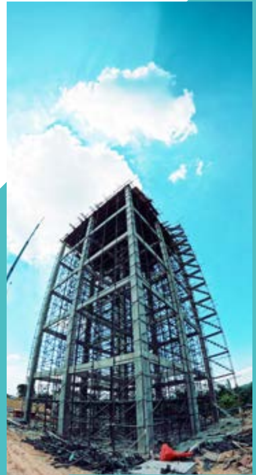
Falsework for Water Tank Construction
